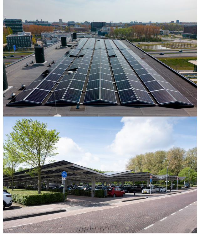
Image 9. Rooftop Solar(top) and Solar Canopy (bottom)
