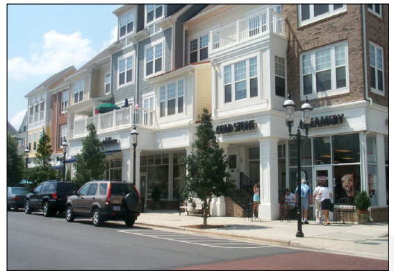
Image 2. Mixed use building with retail and residential
